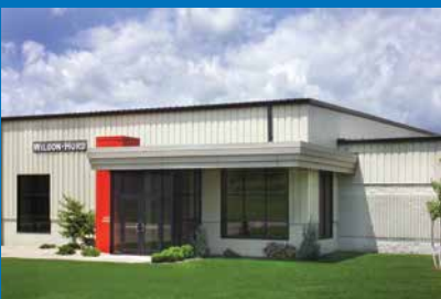
Berlin, WI Advanced Technology Facility
