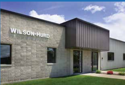
Berlin, WI High Volume Manufacturing Plant
